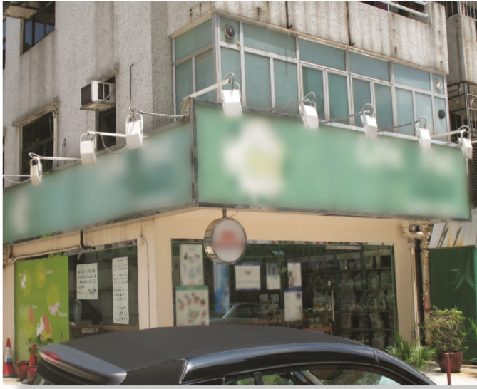
Figures 9 and 10: Examples of UBWs that can be reported under the Reporting Scheme (the left shows a signboard mounted on the external wall; the right shows an unenclosed rooftop structure)
