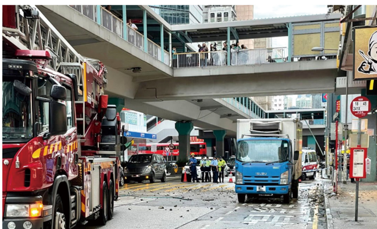
Figure 5: Incident of fallen concrete from the external walls of buildings
